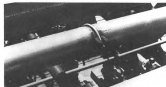
Fig. 2 External clamping used to stop leaks
