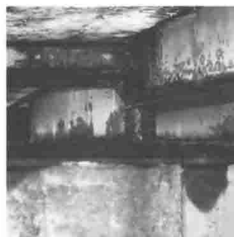
Fig. 5 Corroded regions on a painted highway bridge. Courtesy of R.H. Heidersbach, California Polytechnic State University
